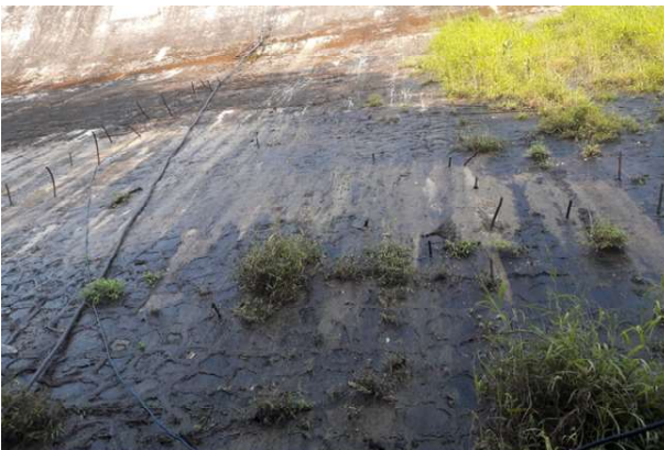
Downstream view of dam before and after preliminary grouting
