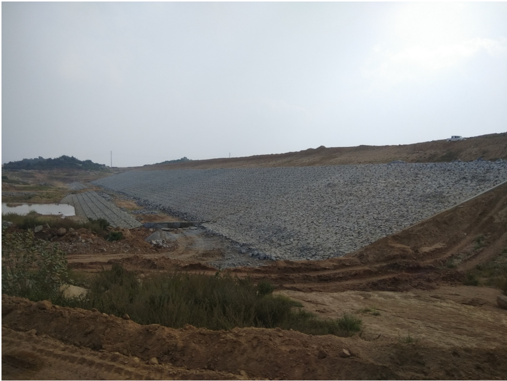
Kurumurthiraya earthen dam
