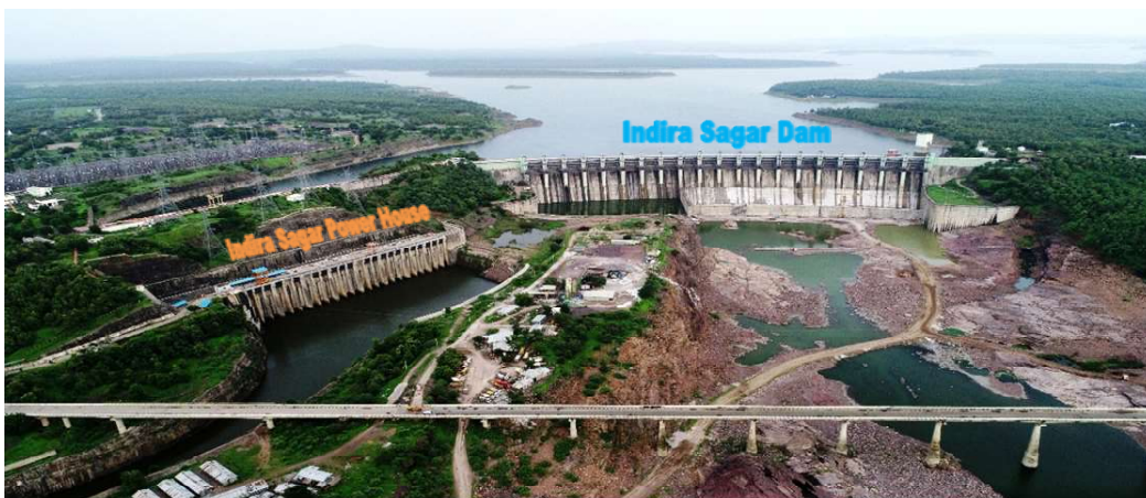
Panoramic View of Indira Sagar Power House with Dam
