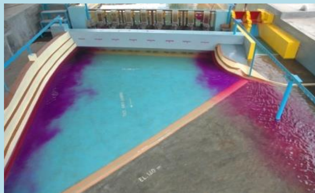
Tailrace Channel, Omkareshwar Project, M.P.
