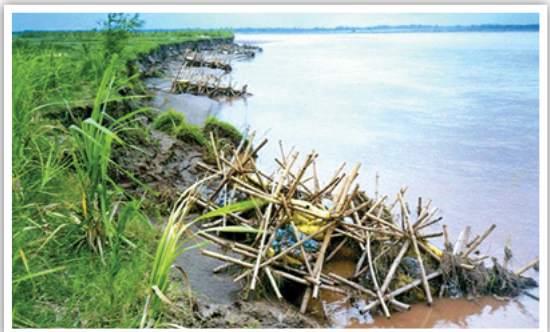
Permeable Porcupine Spur
