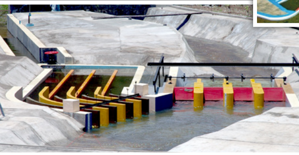
Physical Model of Tapovan Vishnugad hydropower project
