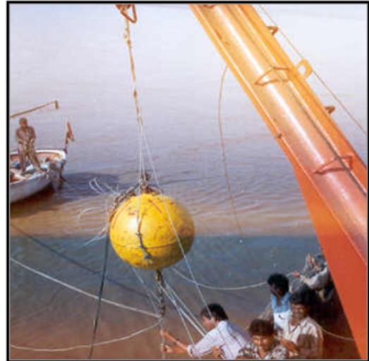
Wave Rider Buoys installation
