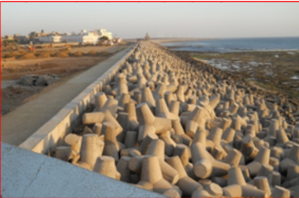
Seawall With Tetrapods at Dwarka
