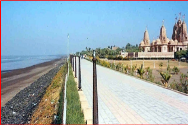
Seawall With Stone Filled Gabions at Tithal
