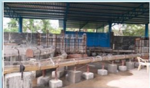
Tailrace Tunnel Punatsangchhu II, Bhutan
