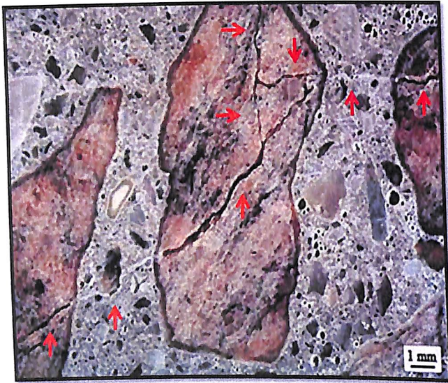
Cracks propagated from one aggregate to other through cement paste (Arrow indicates presence of crack)
