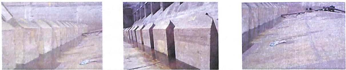
Fig. 16 – Areas repaired in 1994
