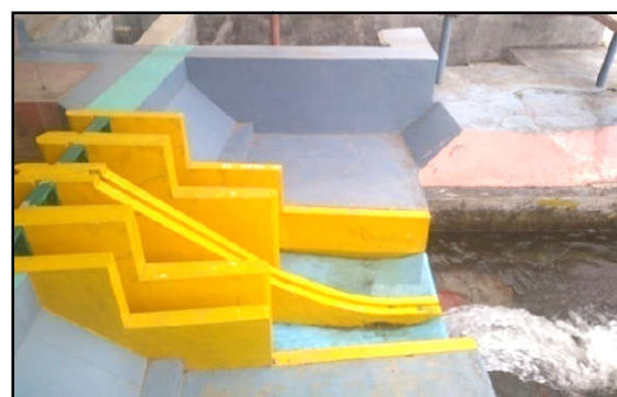
Flow conditions downstream of spillway for Q = 400 \text{ m}^3/\text{s} at MDDL El. 1730.5 m (Gates S3, S4 operating partially)
