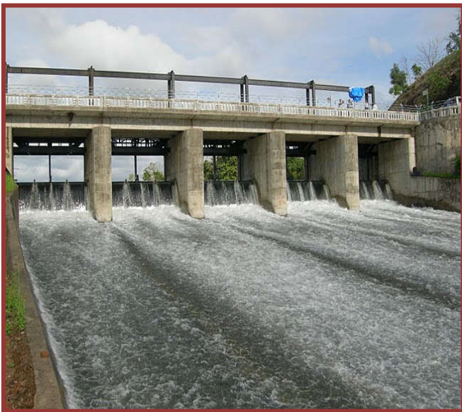
Godbole Gate at Sardar Sarovar Dam
