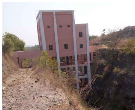
Inspection path LIS Pump house
