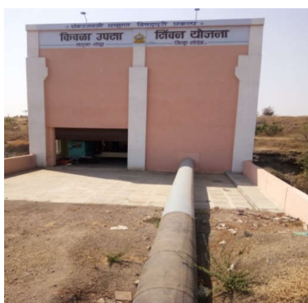
Service road LIS Pump house
