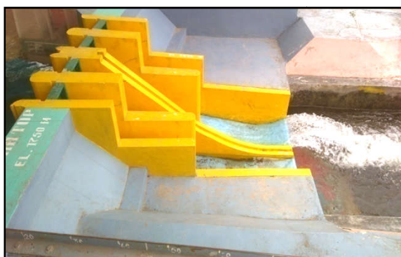
Flow conditions downstream of spillway for Q = 400 \text{ m}^3/\text{s} at MDDL El. 1730.5 m (Gates S1, S2 operating partially)
