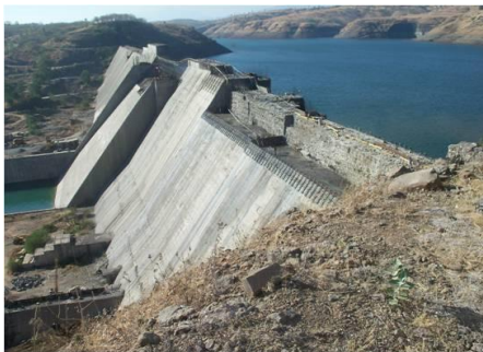
Nilwande dam construction in progress
