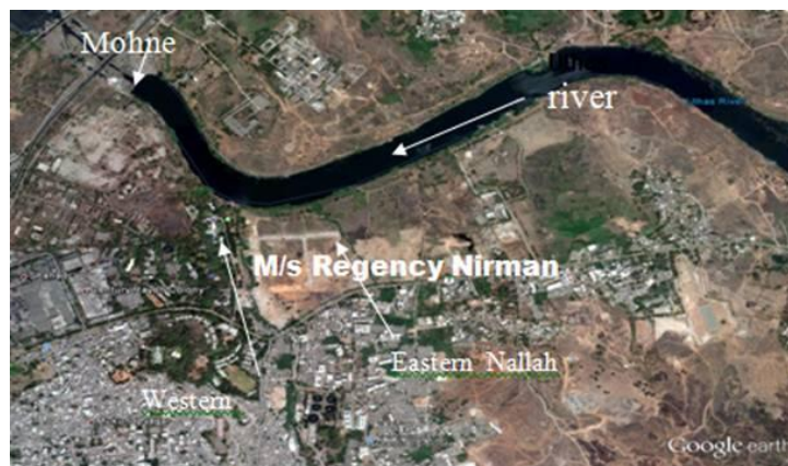
View of site of M/s Regency Nirman Ltd. near Ulhas river
