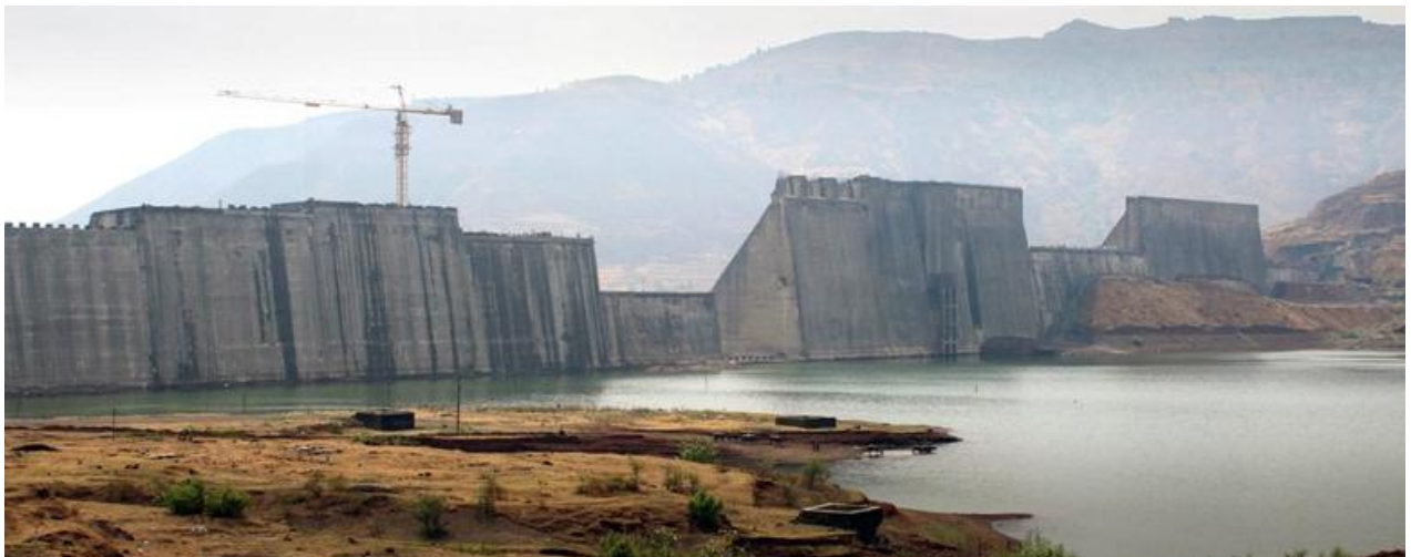
Upstream view of Tarali Dam
