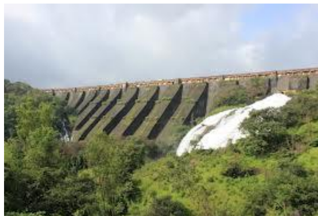
General view of Bhandardara dam
