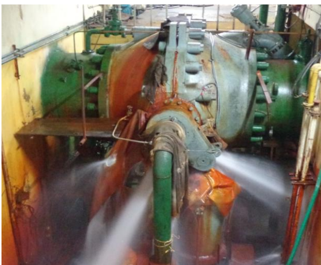
Site conditions at Kopili HEP due to acidic contamination in the reservoir
