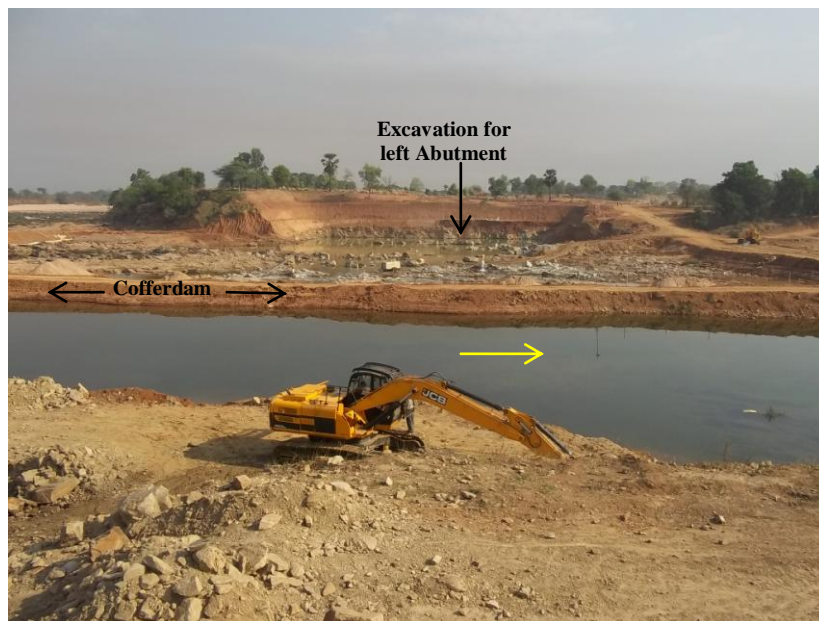
Excavation for left abutment of Kharkai barrage
