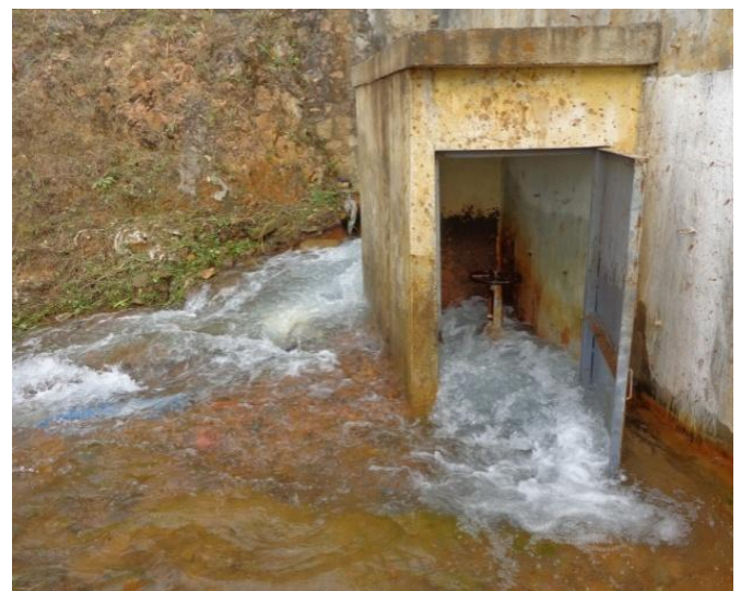
Site conditions at Kopili HEP due to acidic contamination in the reservoir
