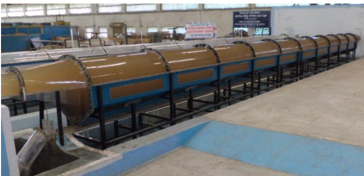
View of desilting Chamber
