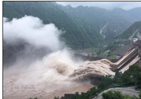
Sediment-laden flow over Salal dam spillway, J&K
