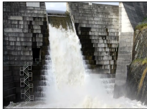
Typical view of stepped spillway
