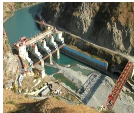
View of the dam site
