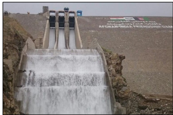
View of the dam site
