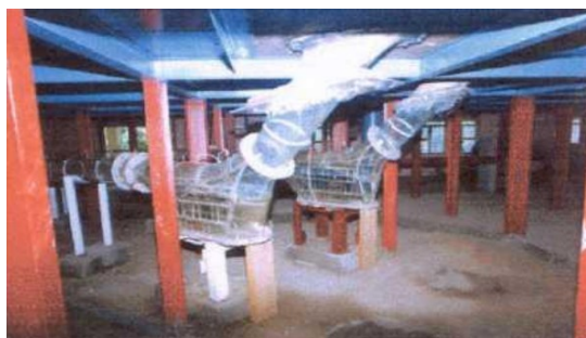
View of the muck pit
