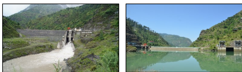
View of the dam site
