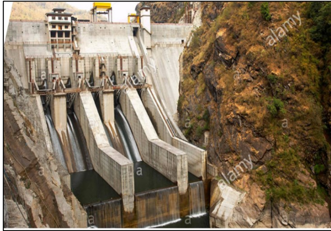
View of the dam site
