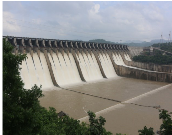
View of the dam site
