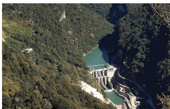
Dams in the narrow valley-Mangdechhu HE Project, Bhutan
