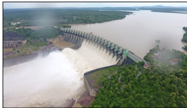
View of the dam site
