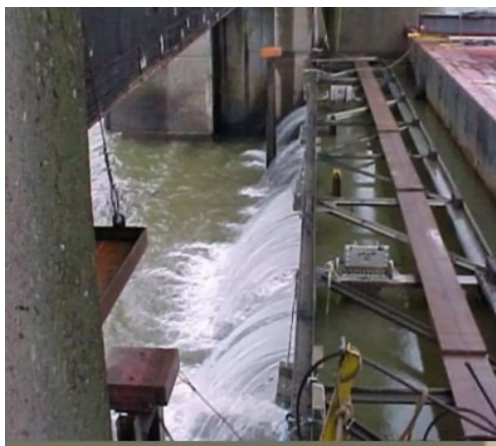
Ogee crest control
