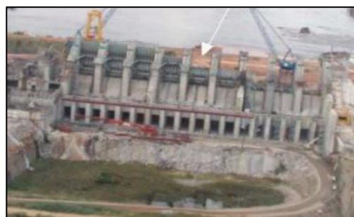
Typical plunge pool of Caruachi HE project
