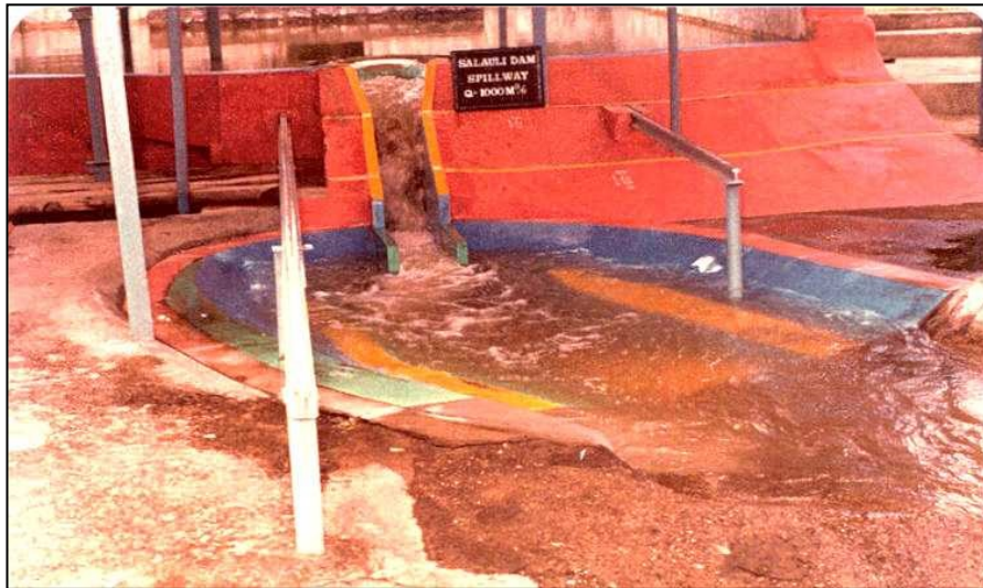
Flow condition in duckbill spillway
