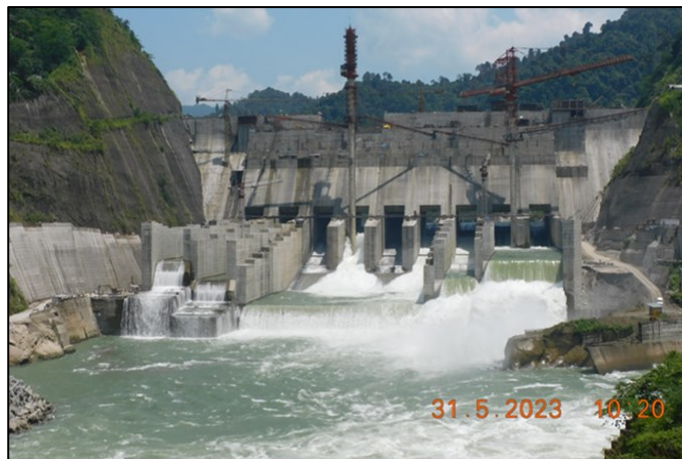
View of the dam site
