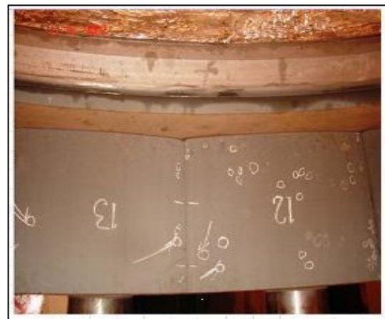
d) Coated guide apparatus (new) assembled at site
