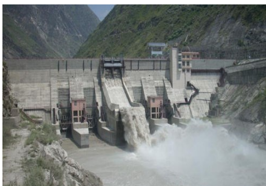
View of the dam site
