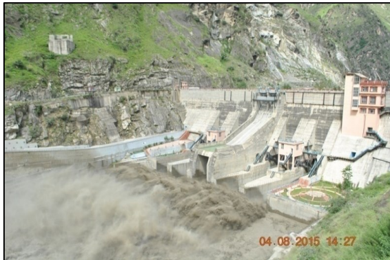
Sediment-laden flow over Nathpa Jhakri dam spillway, H.P.
