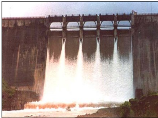
Self-aeration on spillway surface
