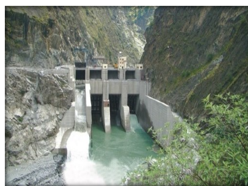
View of the dam site
