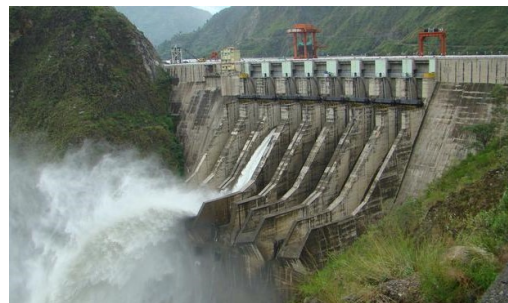
View of the dam site
