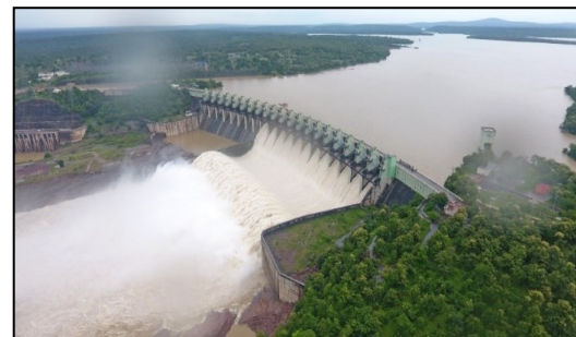
Typical view of overflow spillway
