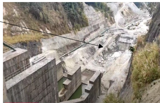
Plunge pool in the dam site
