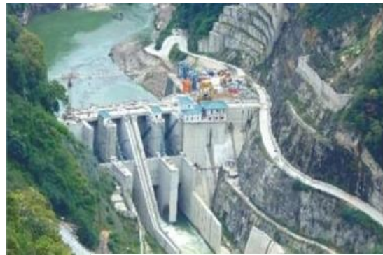
View of the dam site
