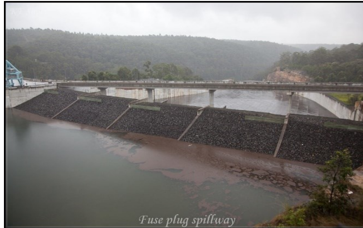
Typical view of fuse plug spillway
