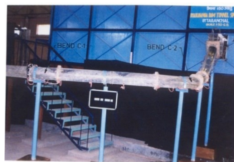
Typical view of tunnel spillway
