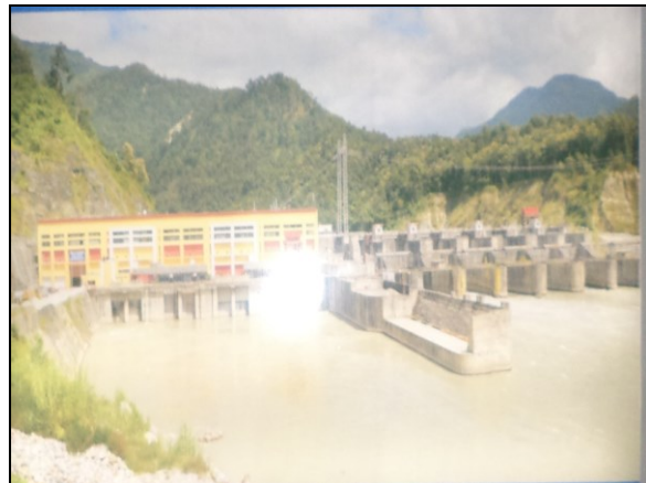
View of the dam site
